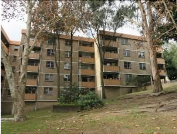
Picture 3 – Open landscaped space showing areas of exposure on slopes
